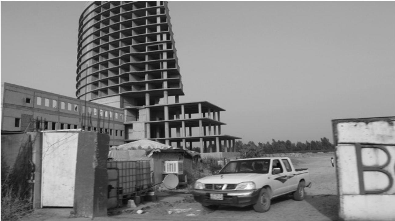
Figure 4.6 Refugees living at a hotel construction site near the Dream City
