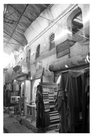
FIGURE 3. EASTERN *QAISARIYA*, TAILORS' WORKSHOPS ALONG THE EASTERN HALLWAY UNDER A TEMPORARY SHELTER WHICH REPLACED THE COLLAPSED BARREL VAULT, ALSO THE WOODEN GALLERY IS MISSING AND THE UPPER-FLOOR ROOMS ARE NOT ACCESSIBLE ANY MORE (2012, TU BERLIN/DAI, D. KURAPKAT).
