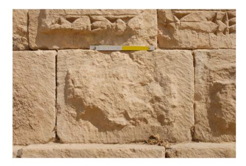
FIGURE 4. CHISEL MARKS ON THE OUTER BANDS OF A BLOCK (PHOTO BY M. GATTI, © MAIA).
